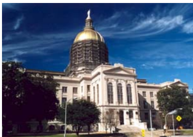
Georgia state capitol building.
